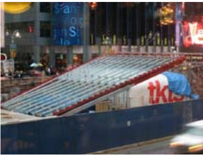
Figure 2 The complete structural chassis, prior to fixing of cladding
