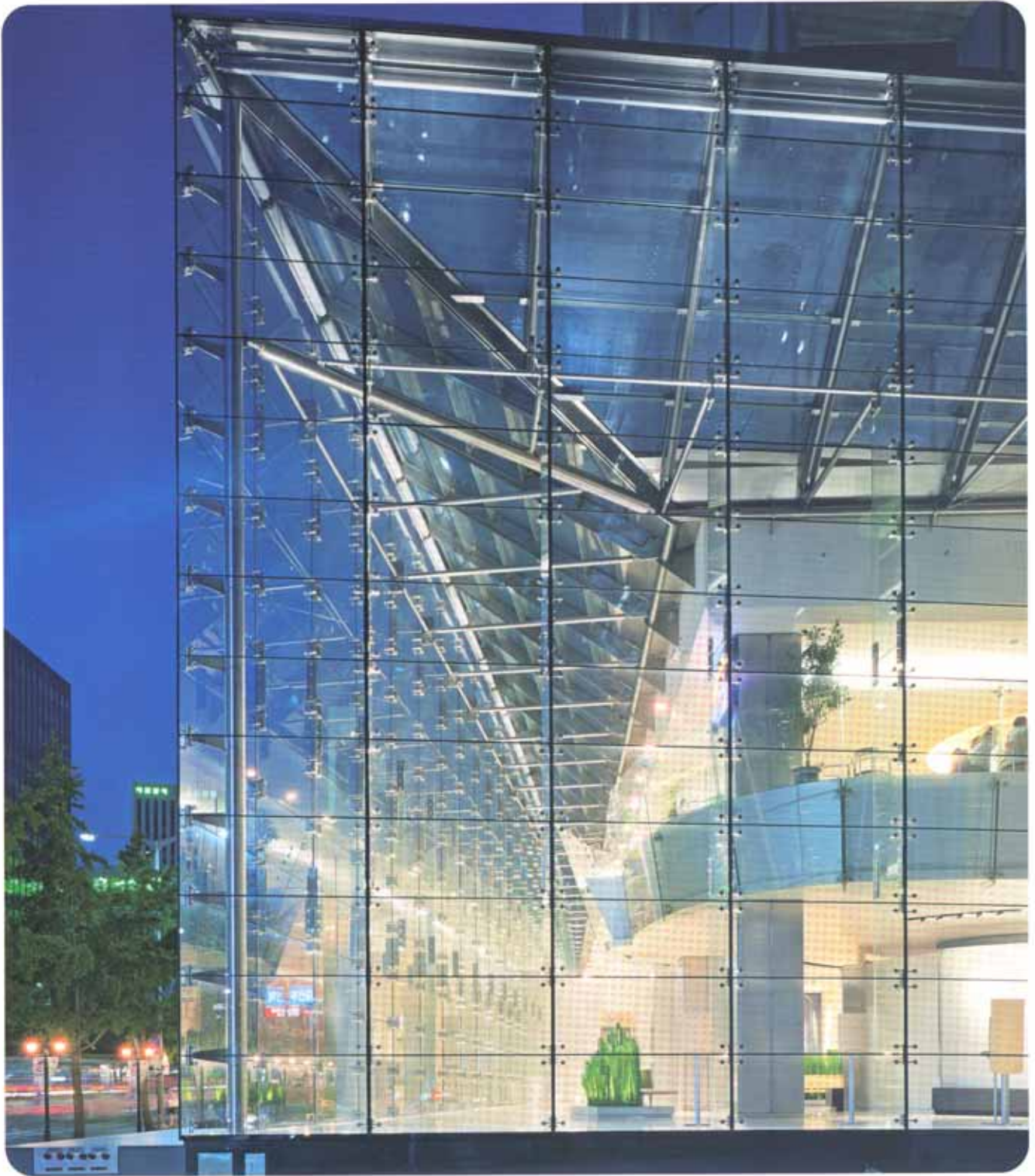
Samsung Headquarters Renovation, Seoul-Korea, Arch.: Kohn Pedersen Fox Associates PC-New York
